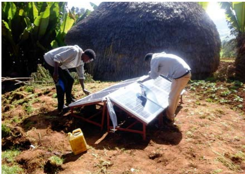
Solar installation in Laka
